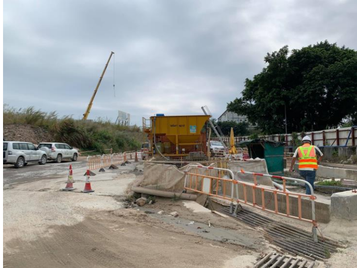
Q6: Wastewater treatment facility 24 cu. m.
