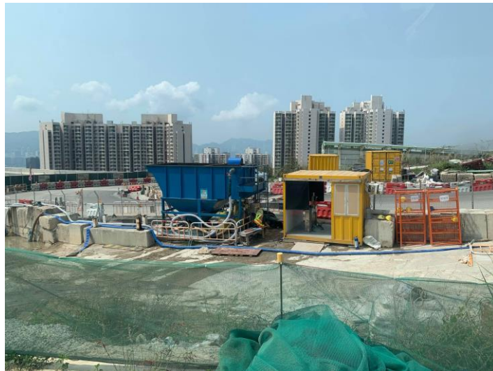
Q4. Wastewater treatment facility Temporary Water Reservoir 150 cu.m + AquaSed of 60 cu.m per hour
