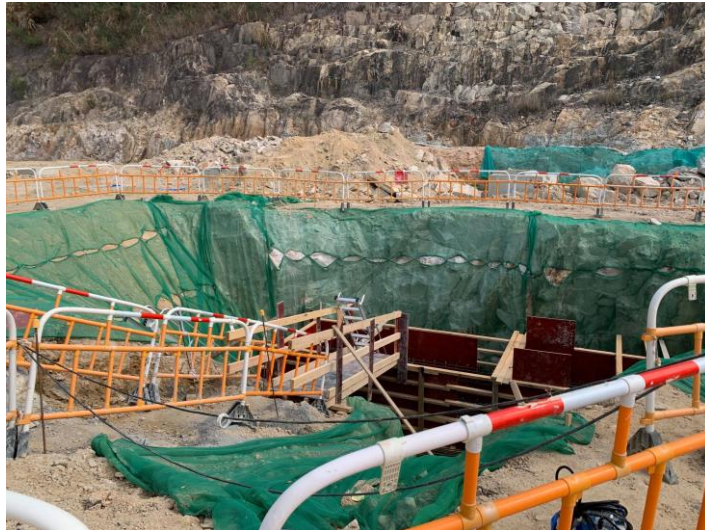
Impermeable cover for slope at Cavern.
